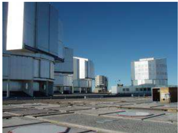
The four domes of the Very Large Telescope of the European Southern Observatory (ESO), installed on the Paranal Mountain in Chile. Each dome contains a 8.20m diameter telescope. © DP
